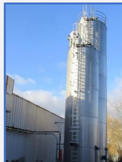
Silo alu 27 000 LITRES Aluminium sugar silo
